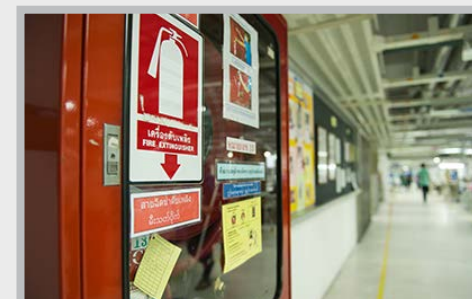
Fire safety equipment in our Thailand factory
