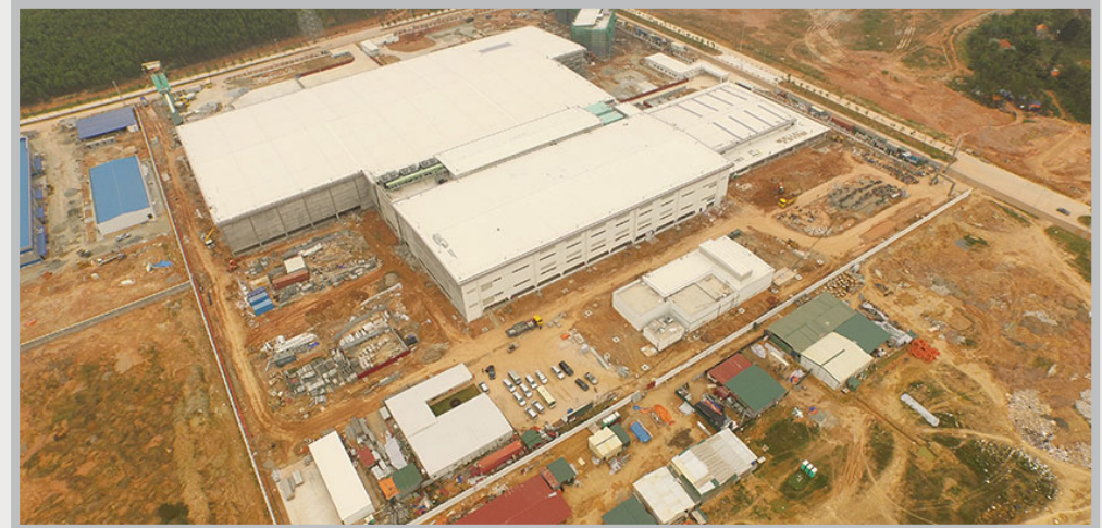
Construction underway at VNG
