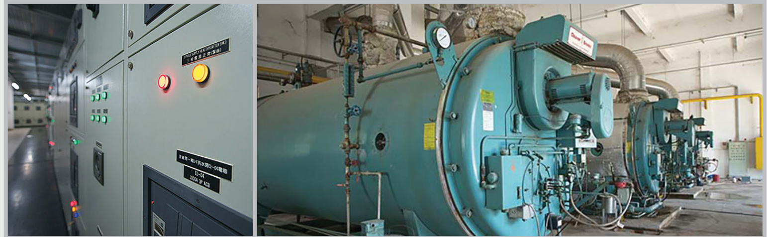
Energy-efficient equipment inside our factory in Dongguan
